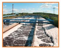
The traditional approach is to dose anti-foam into the process on a continual basis. This dose rate is typically set to cope with foam during the plant's peak demand. However on average this is far too high and in some systems there is little or no foam generation for most of the time. Alternatively the addition of chemicals is often done randomly, in far too large quantities and too late. This reactive
